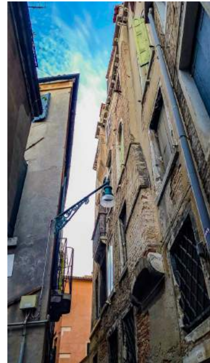
Rhythm Between Walls Narrow by design, these streets offered protection, nurtured connection and moved to the quiet rhythm of survival.
